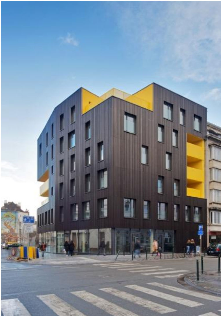
AR : B12 – EG : Gillion Construct
