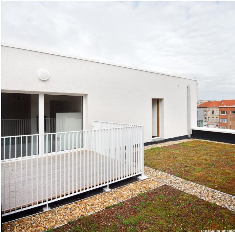
AR : K2A – EG : Gillion Construct
